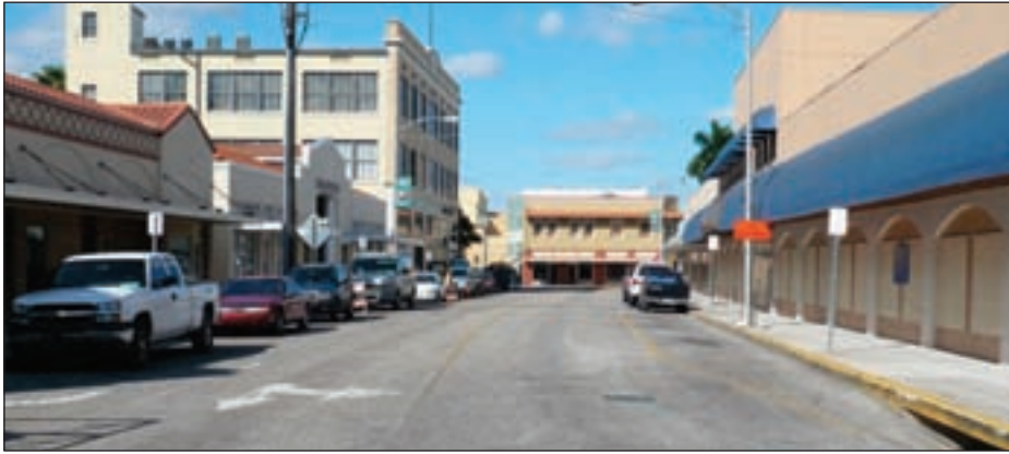
Broadway before streetscape project
